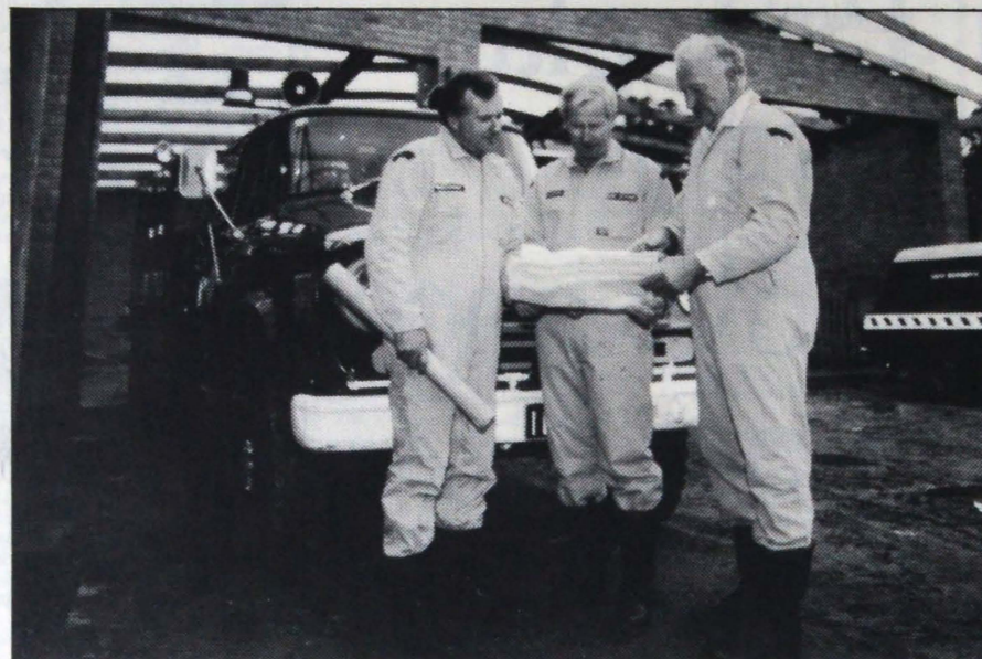
Les Reid (at right) in uncharacteristic pose during the building of the South Warrandyte Fire Station. Les was usually wielding a shovel or a hammer or doing something about the place. On Les's left is ex captain Kirk Ritchie and captain John Haddon.
