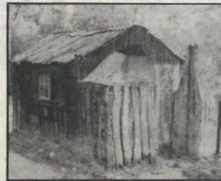
The historic cottage - as it was before the cover was erected.
