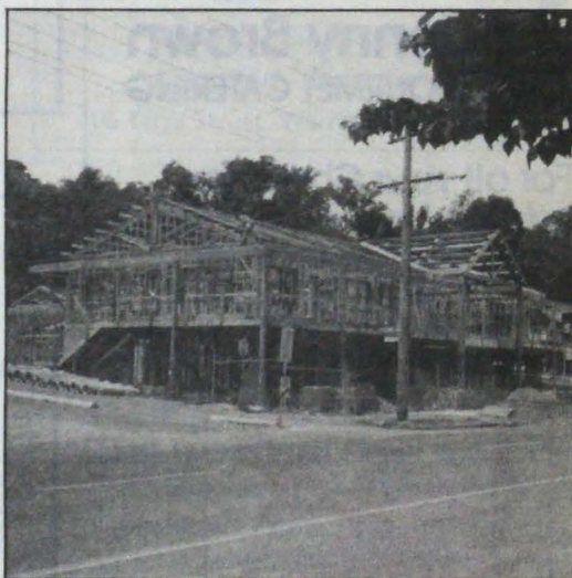
Above: Our new community centre — reality in timber and brick
