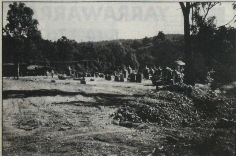
Land cleared by the bulldozer
