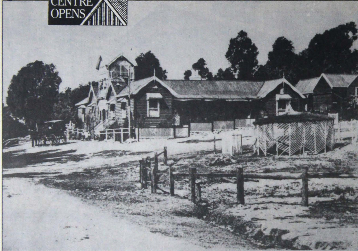
The Mitchell Avenue-Yarra Street corner. The community centre site was vacant at this time. Beyond is the Warrandyte Hotel, which burnt down in 1925. It helped inspire the design of the new centre.
