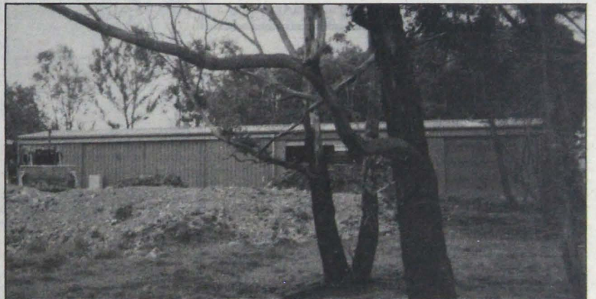
Work continues on the hazardous chemicals facility at Pound Bend.
