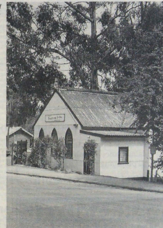
The newly renovated Gospel Chapel.
