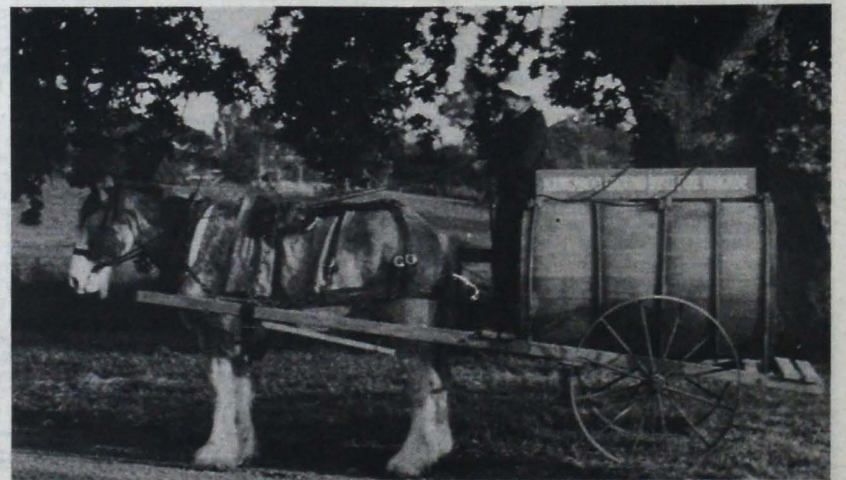
Replica of the fire cart built for the Kangaroo Ground Fire Brigade in 1914.
