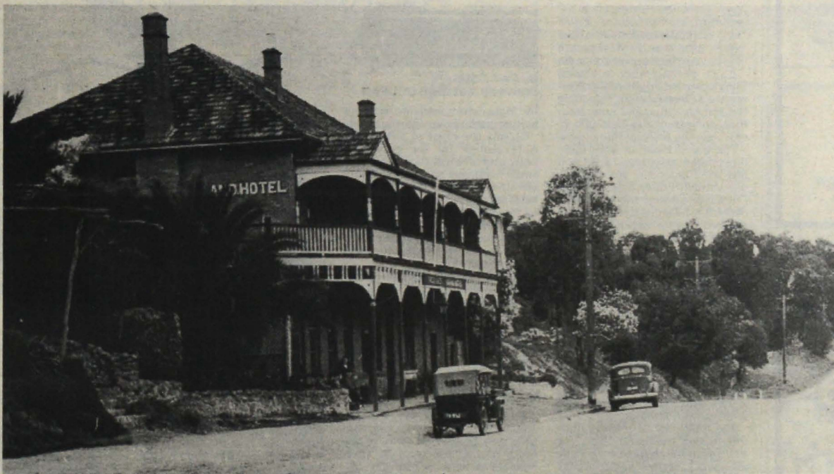
The middle years: Framed in its environment by local stonework, its own garden and the returning roadside bush.
