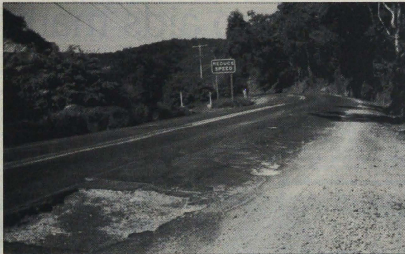
Soft edges and potholes make Research Road dangerous. (Pictures by Jan Tindale)
