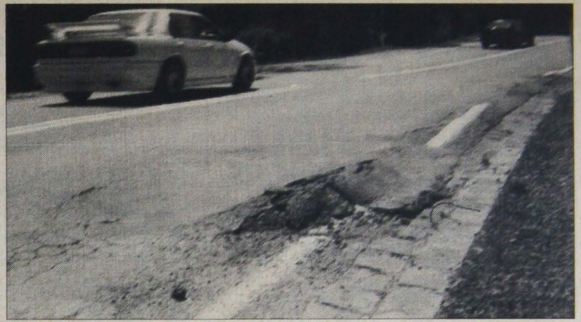
Patches last only until the next rain on roads with heavy traffic.
