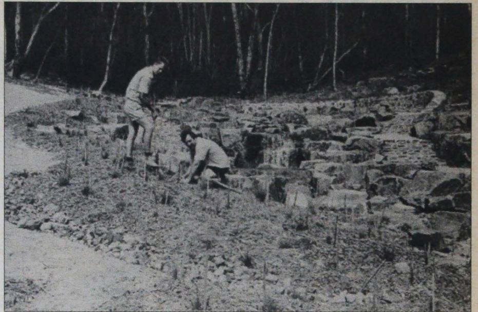
Works manager, Alan Bellinger, right, and staff member, Chris Walshe, plant out the newly opened waterfall at the Andersons Creek Cemetery.
