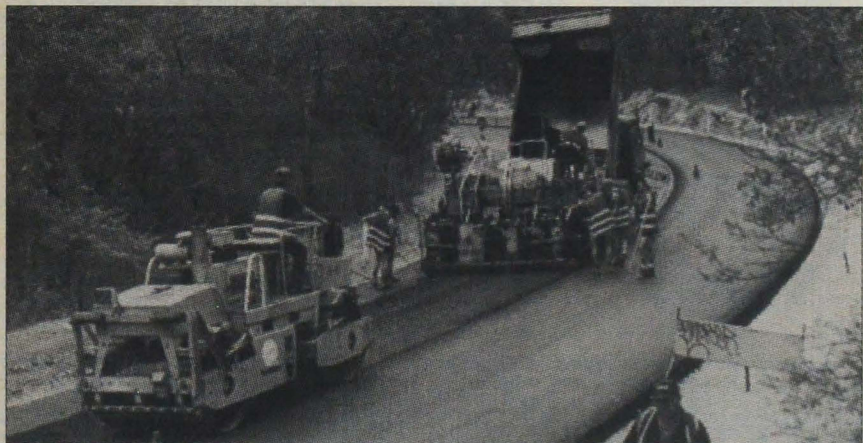
Work proceeding on Melbourne Hill. (Picture by Clinton Grybas)
