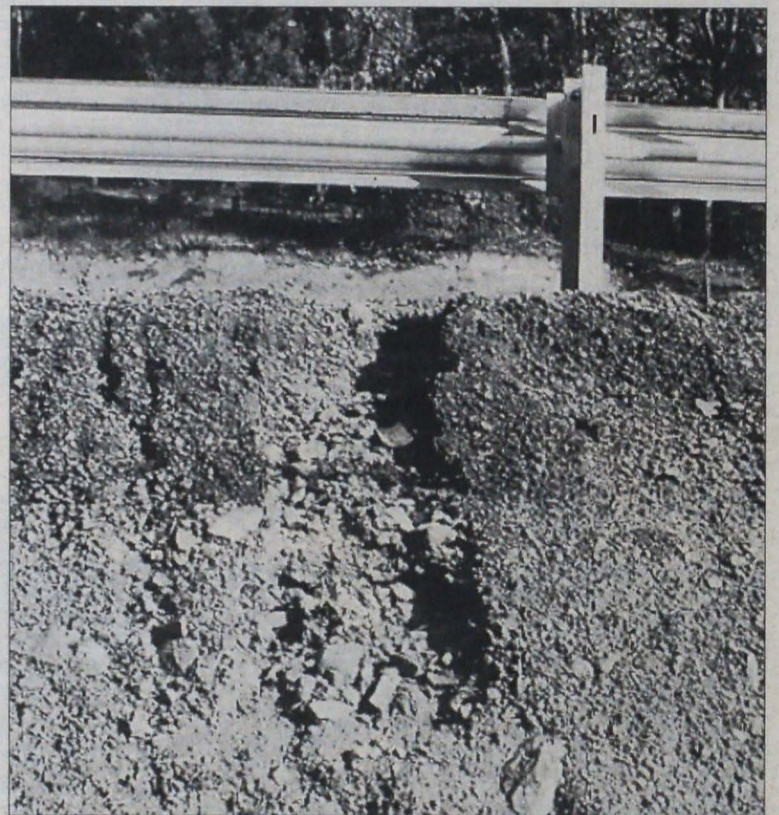
The bitumen surface is breaking up (above) and severe erosion is damaging fill (below and right) on the Ringwood Road. (Pictures by Jan Tindale)
