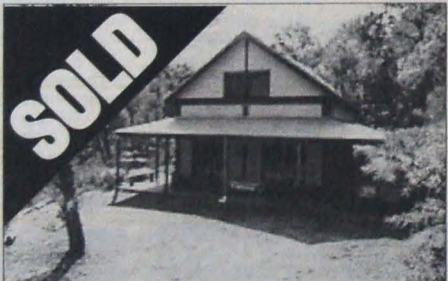
15 Hillcrest Road, Hurstbridge
