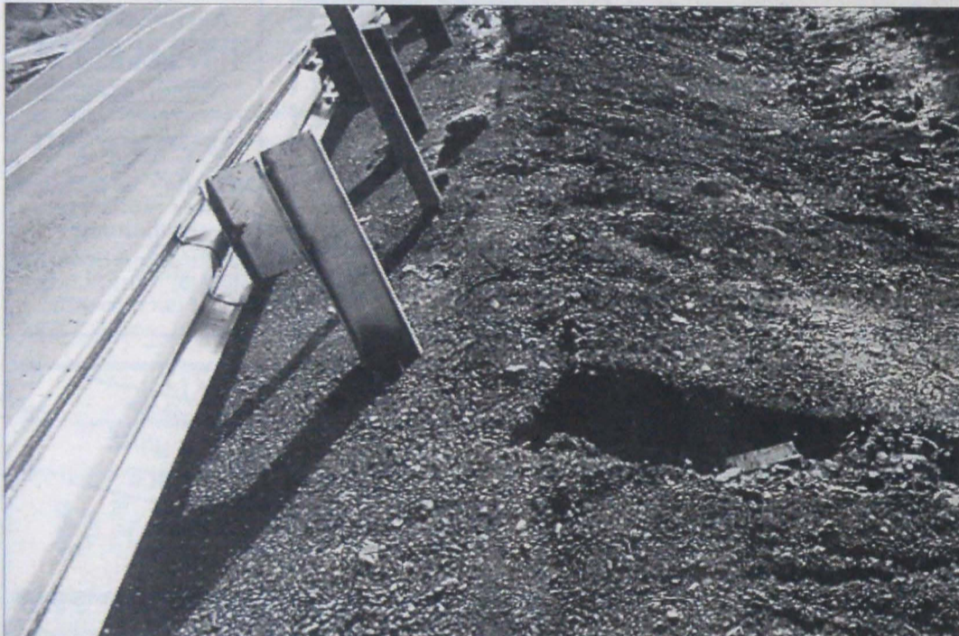
The bitumen surface is breaking up (above) and severe erosion is damaging fill (below and right) on the Ringwood Road. (Pictures by Jan Tindale)
