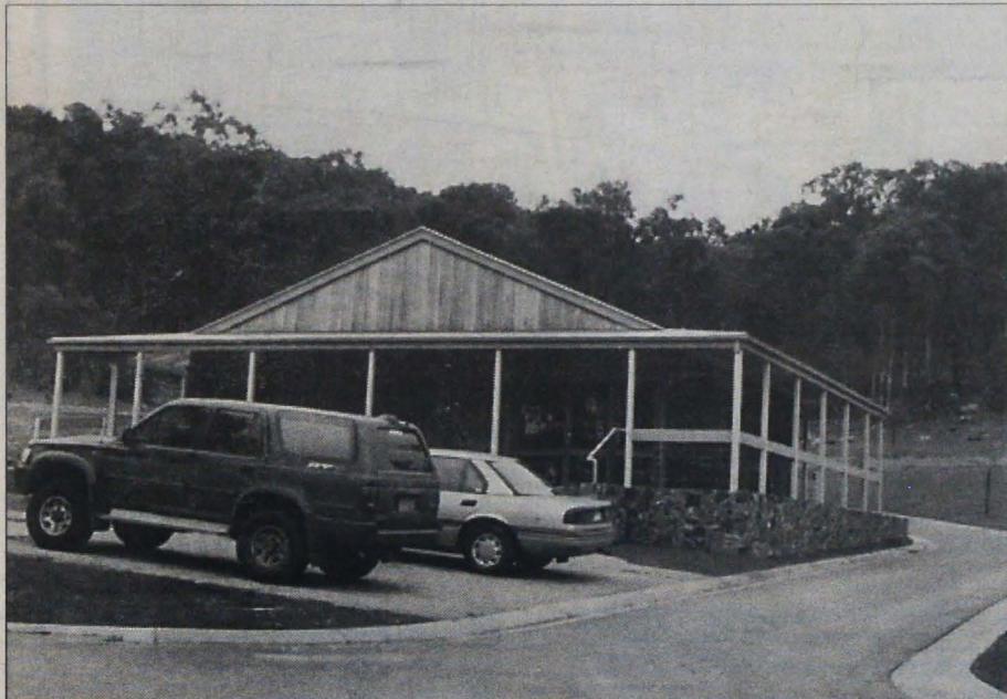
The new office at Andersons Creek Cemetery.
