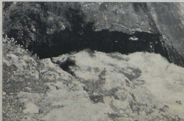
The Tunnel at Pound Bend in flood.
