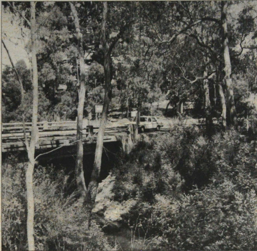
Mullum Mullum Creek bridge crossing Warrandyte Road: is this the spot for a freeway? (Picture by Jan Tindale)
