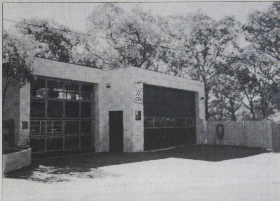
North Warrandyte's fire station. Except it's now in Research. (Picture by Jan Tindale)
