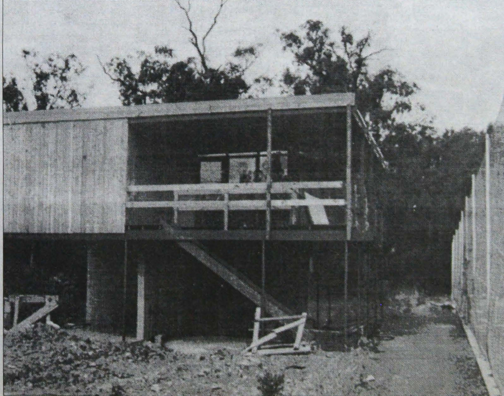
Flashback. Warrandyte Tennis Club's current Taroona Avenue home under construction in 1978.
