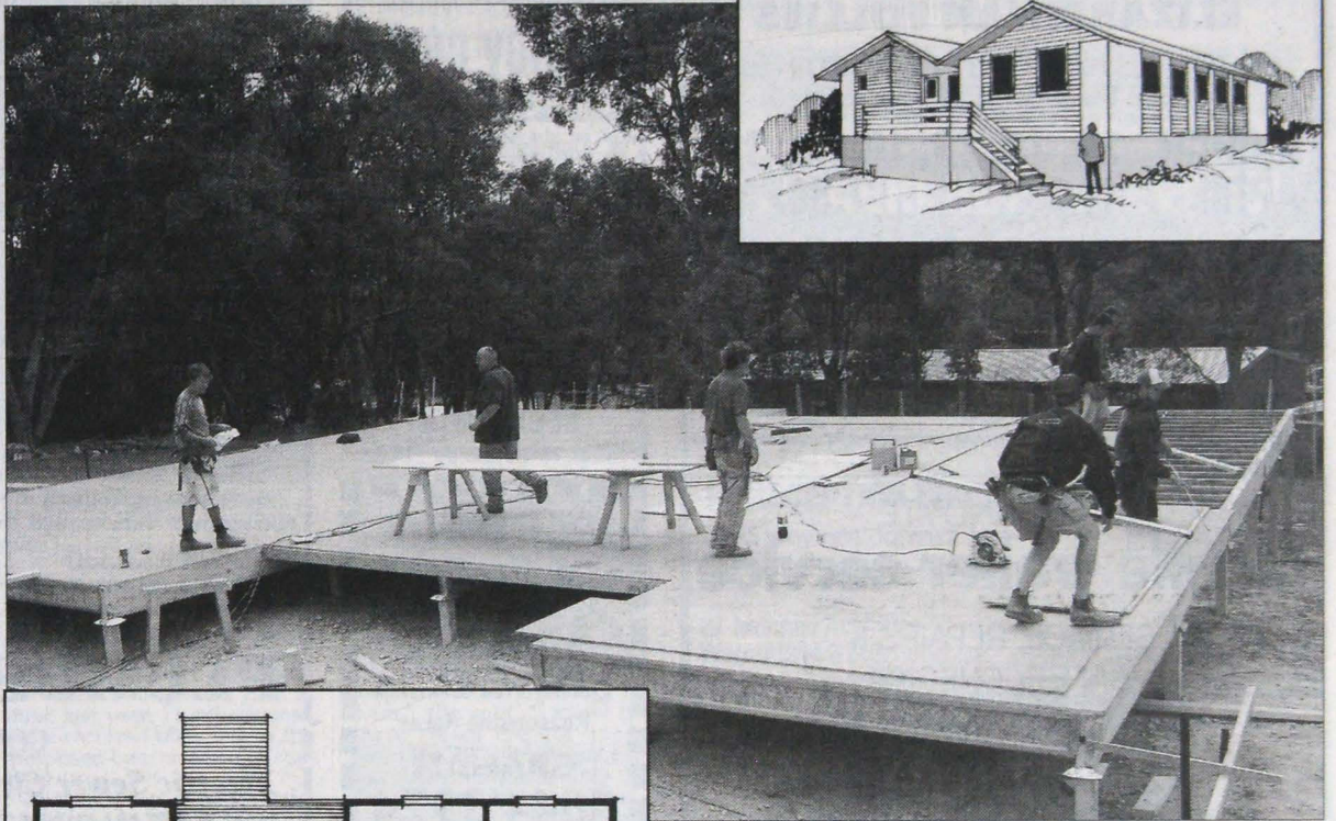
From the ground up: building apprentices from Holmesglen TAFE completing the floor of the new depot offices. (Picture by Stephen Reynolds)
