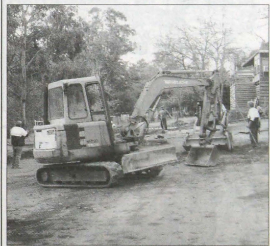
Men at work: new parking bays take shape.
