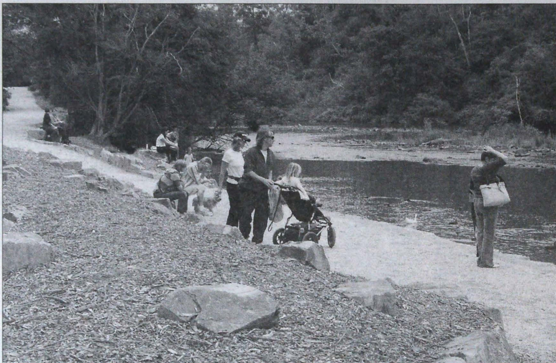
The new riverbank path and stone retaining wall below the bakery is finished and is already proving popular. (Picture by Sandy Burgoyne)
