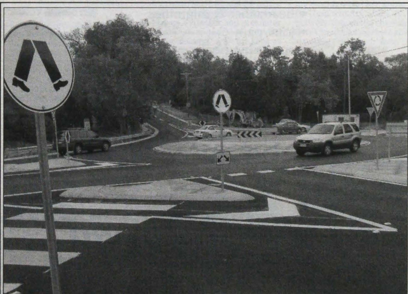
The journey between Warrandyte and Park Orchards has been made safer with the completion of the new $1m roundabout at the intersection of Knees, Stinton and Falconer roads. Built by Manningham council, the project was partly funded through a $362,000 grant from the Federal government. (Picture by Stephen Reynolds)
