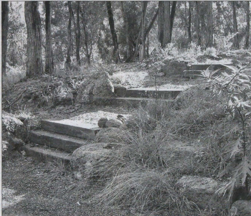
Garden steps can be built of railway sleepers.
