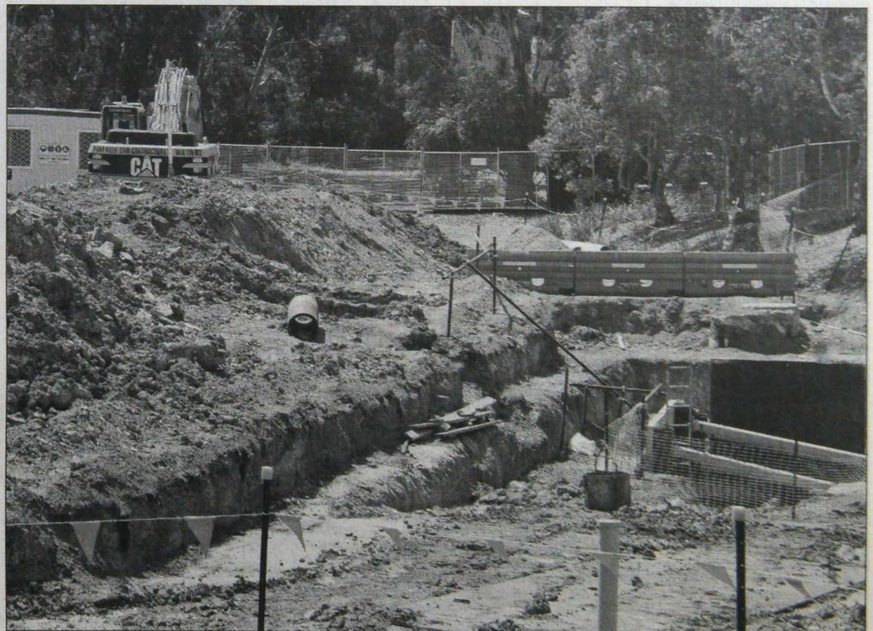
No, it's not a bomb site! Yarra Valley Water is currently carrying out excavation works towards the building of increased emergency storage capacity at the Tarooma Avenue sewerage pumping station next to the second oval. This will reduce the potential risk of sewage overflows into nearby Andersons Creek and, eventually, the Yarra River. (Picture by Stephen Reynolds)
