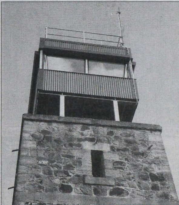
Firespotters cabin sits atop the tower.
