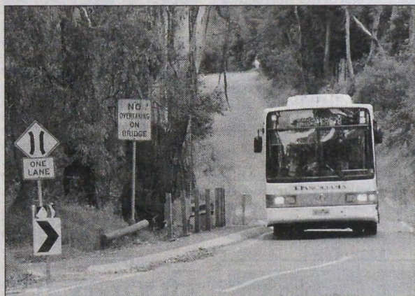
A Panorama bus negotiates the one-lane bridge in Everard Drive.
