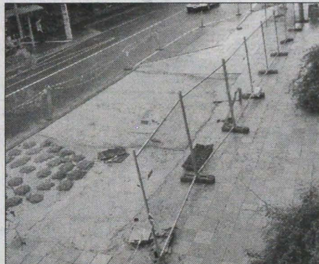
2 Work is abandoned at the community centre.
