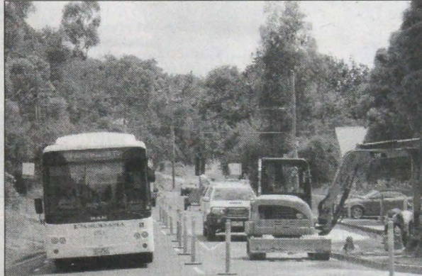
5 Traffic is diverted as Gospel carpark work continues.
