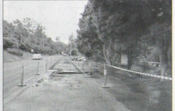
6 Work is abandoned at the Gospel bus bay.
