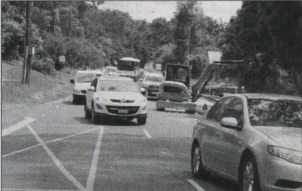
4 Workmen begin removing bus bay at the Gospel carpark.
