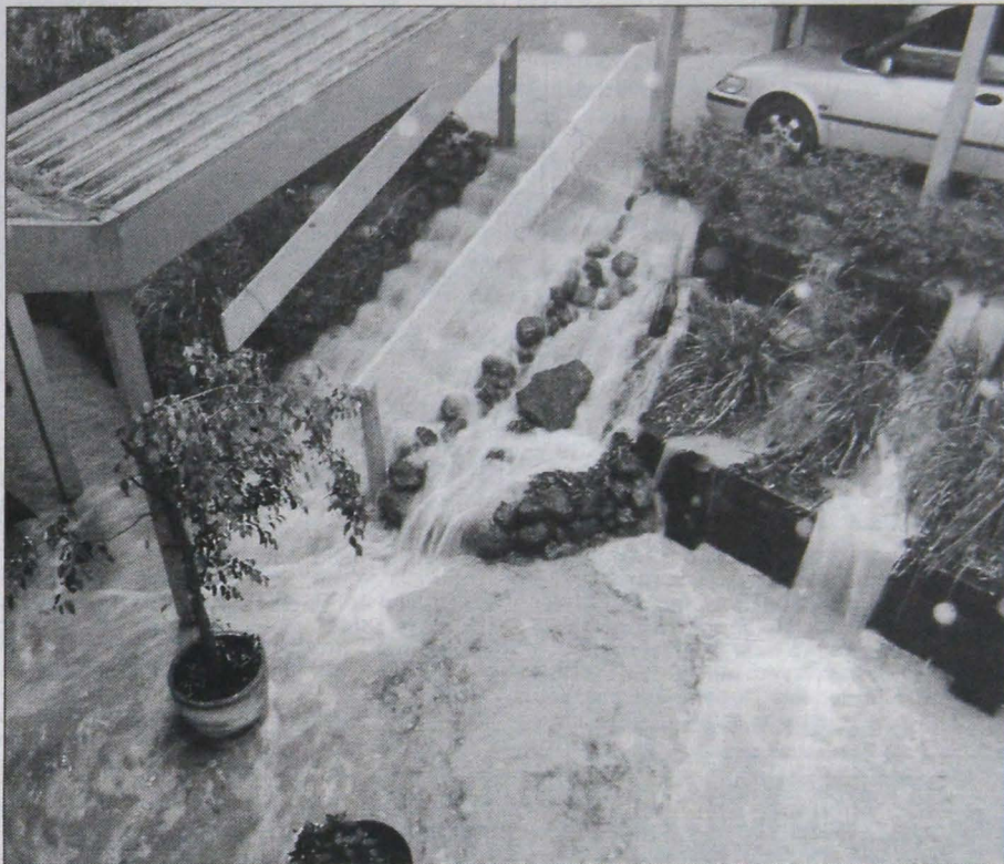
Water, water, everywhere: The Davies' house in Bradleys Lane was inundated.
