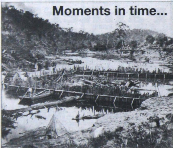
'Coffer Dam on the Yarra' by Carl Walter.
