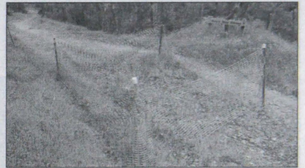
That sinking feeling: Old mining work caused this sinkhole to appear on the Whipstick Gully Track.
