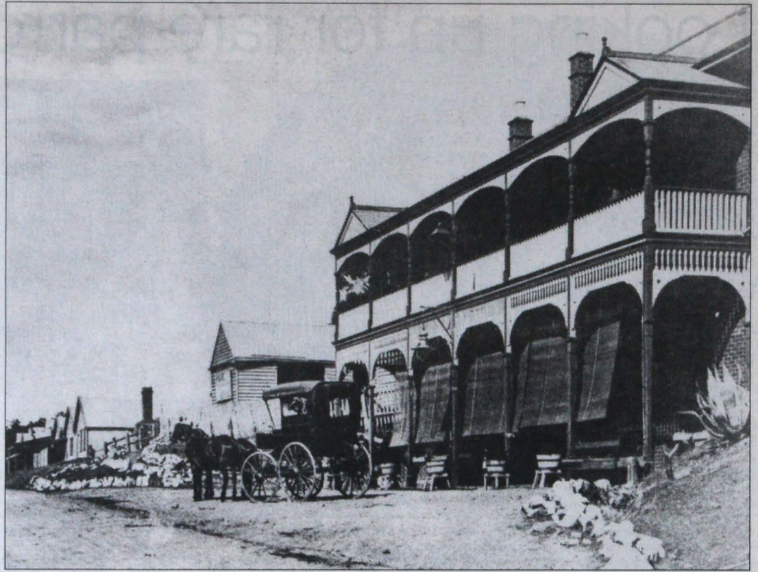
The Grand Hotel (complete with verandahs)
