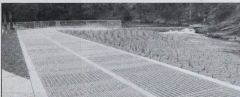
The new fishway.
