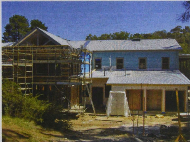
New rear extension on refurbished building.
