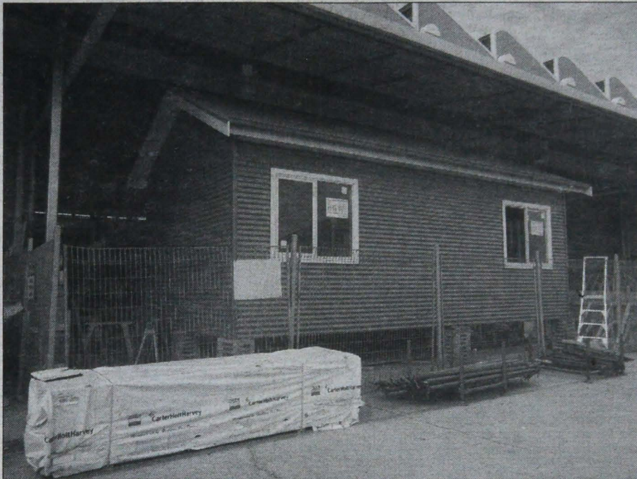
Ready to roll: New FOWSP building at Holmesglen TAFE.
